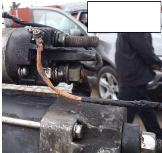
Overheated solenoid wire
