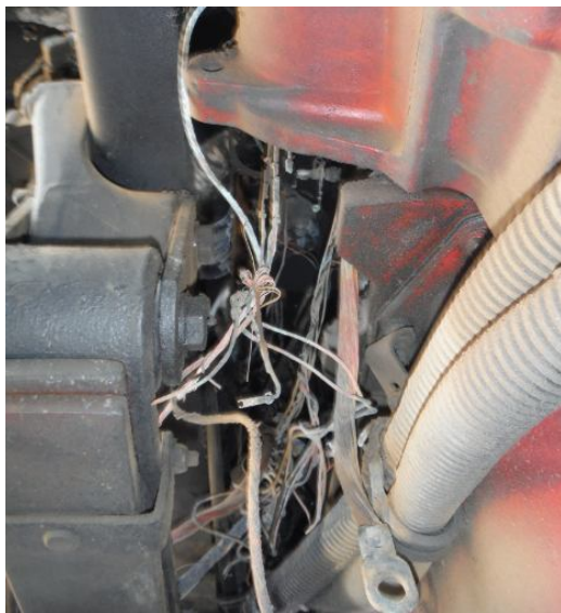
Control wiring around starter
